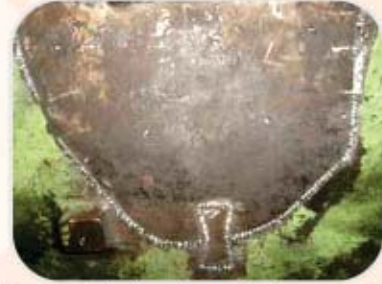
Patch Plate stitched on blown-off portion of Marine Engine by using Dovetail
