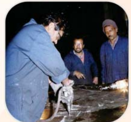
BOTTOM TABLE OF 63/12MN WHEEL FORGE MACHINE UNDERGONE REPAIR AFTER BROKEN
