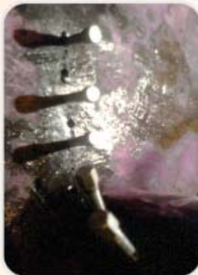
Plug stitching on crack portion
